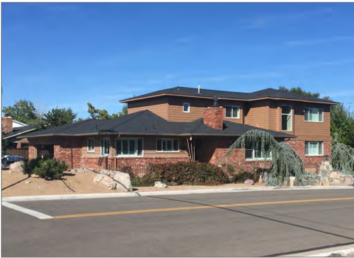
Example: Renovations and additions
