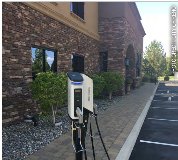
Example: Electric vehicle charging stations
